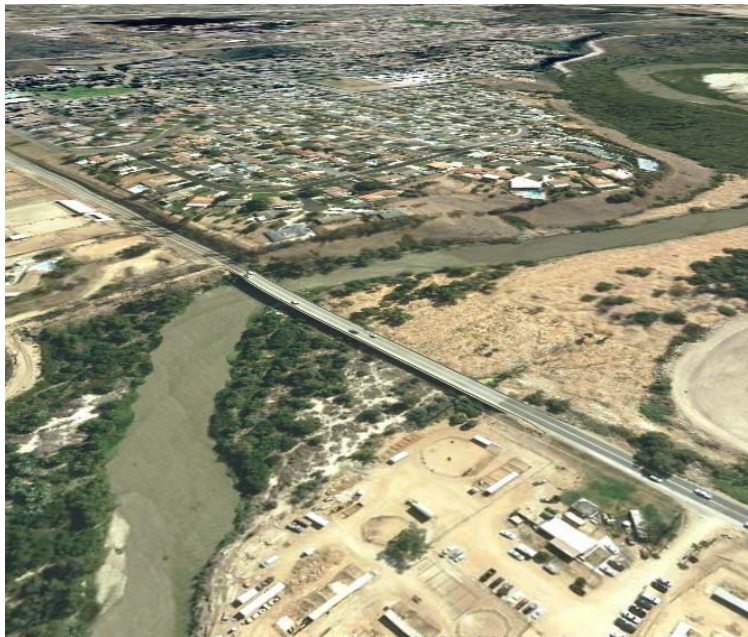
Figure 2-5 Aerial View of the Hamner Avenue Bridge
