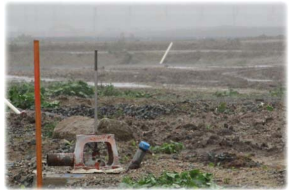
An Abandoned Well on a Property That is to be Developed
