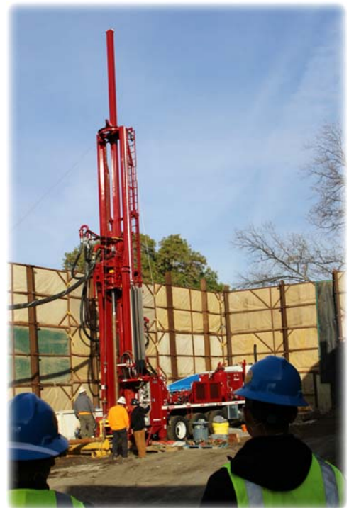
Construction of the Pomona Extensometer
