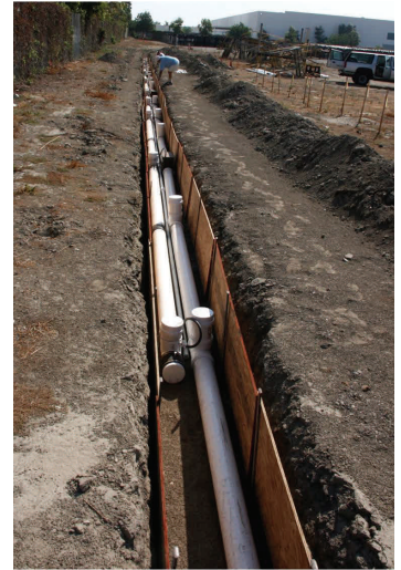
Horizontal Extensometer Construction
