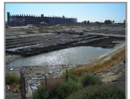
Cleaning Operations—Hickory Basin
