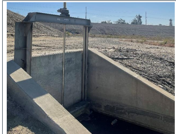
Photo 7 Pump Station Intake Structure
