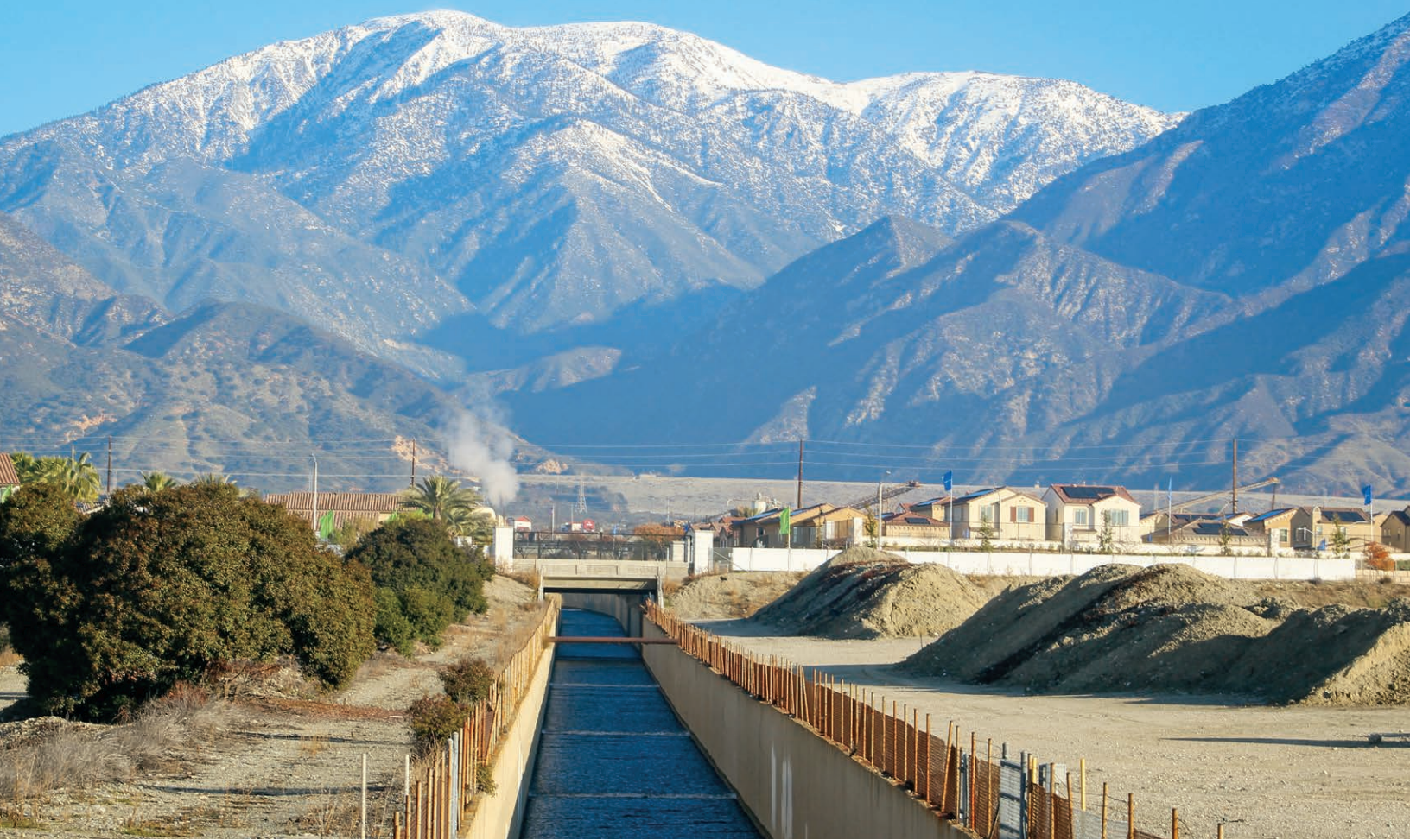
San Antonio Channel runs between two groundwater recharge basins.
