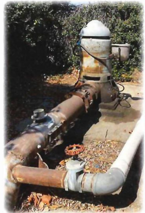
Metered Irrigation Well
