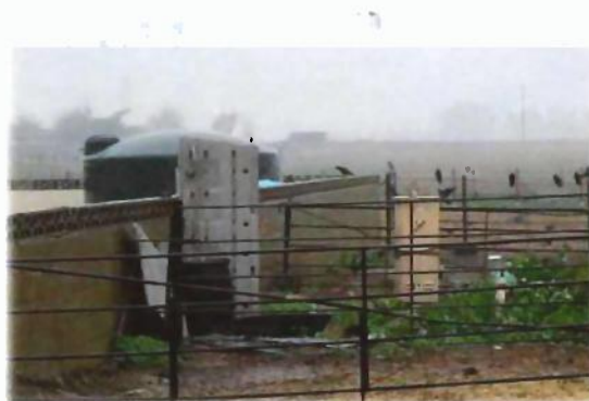
Well Water Replaced by Alternative Supply via Green Tank
