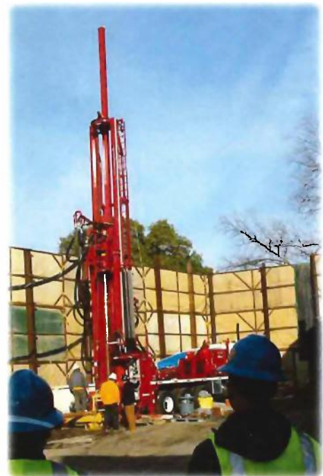
Construction of the Pomona Extensometer
