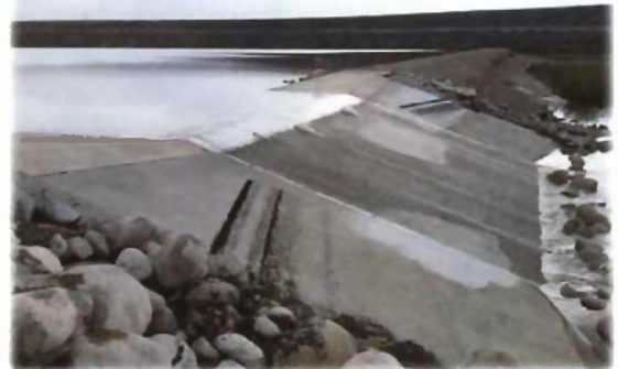
San Sevaine 5 Basin After a Rainstorm in January
