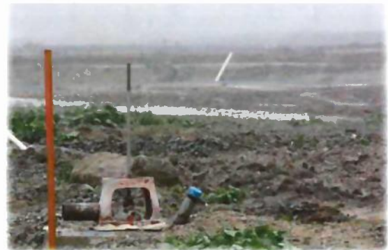
An Abandoned Well on a Property That is to be Developed
