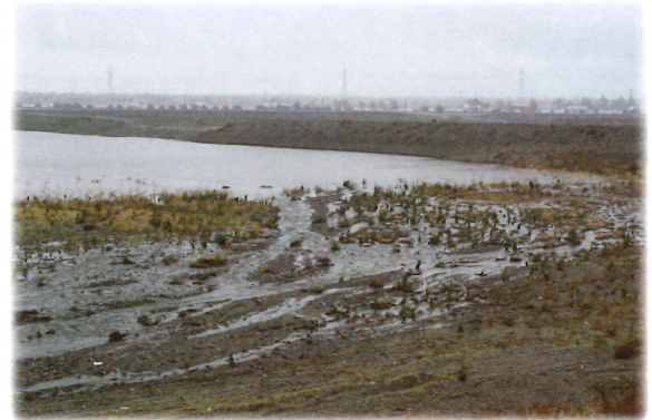
Stormwater Flowing Into San Sevaine 1 Basin
