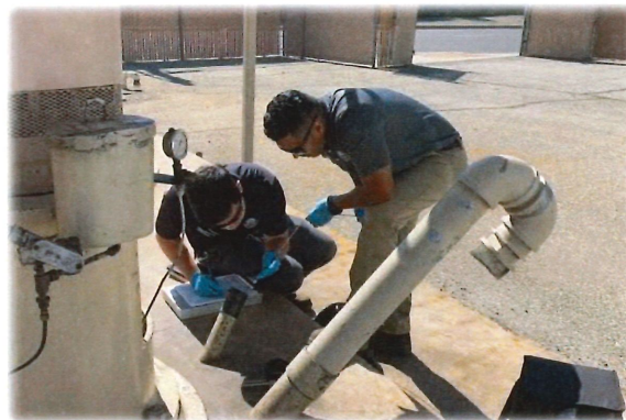
Ops Staff Taking a Groundwater Level Measurement
