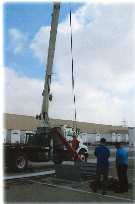
Well Repair at a Water Quality Sampling Site
