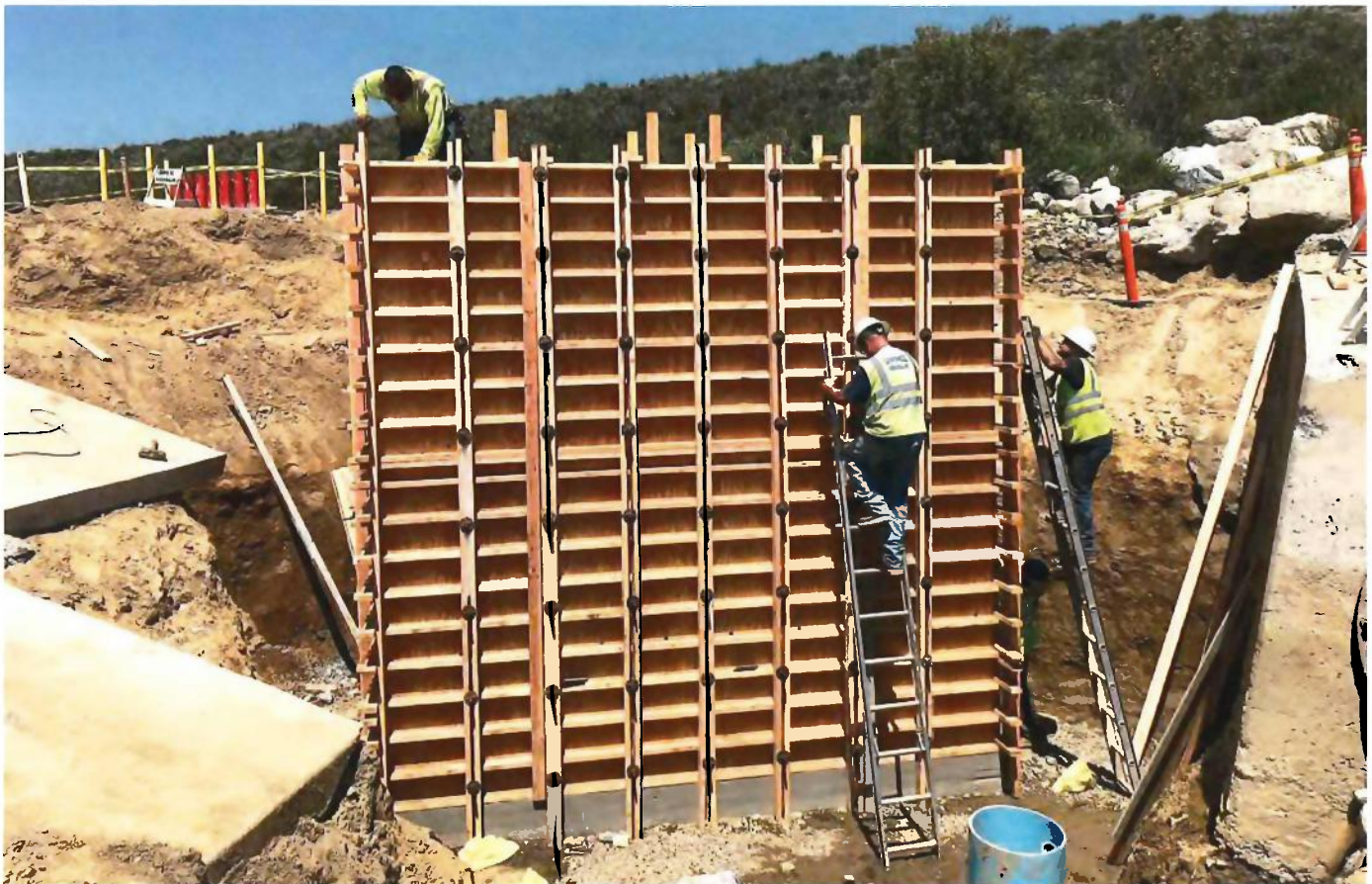
Construction underway at San Sevaine Basin.
