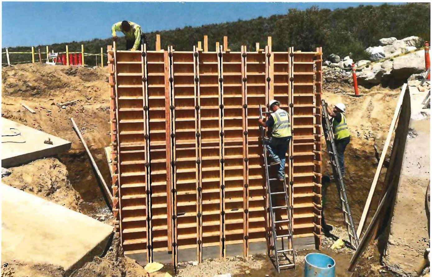
Construction underway at San Sevaine Basin.
