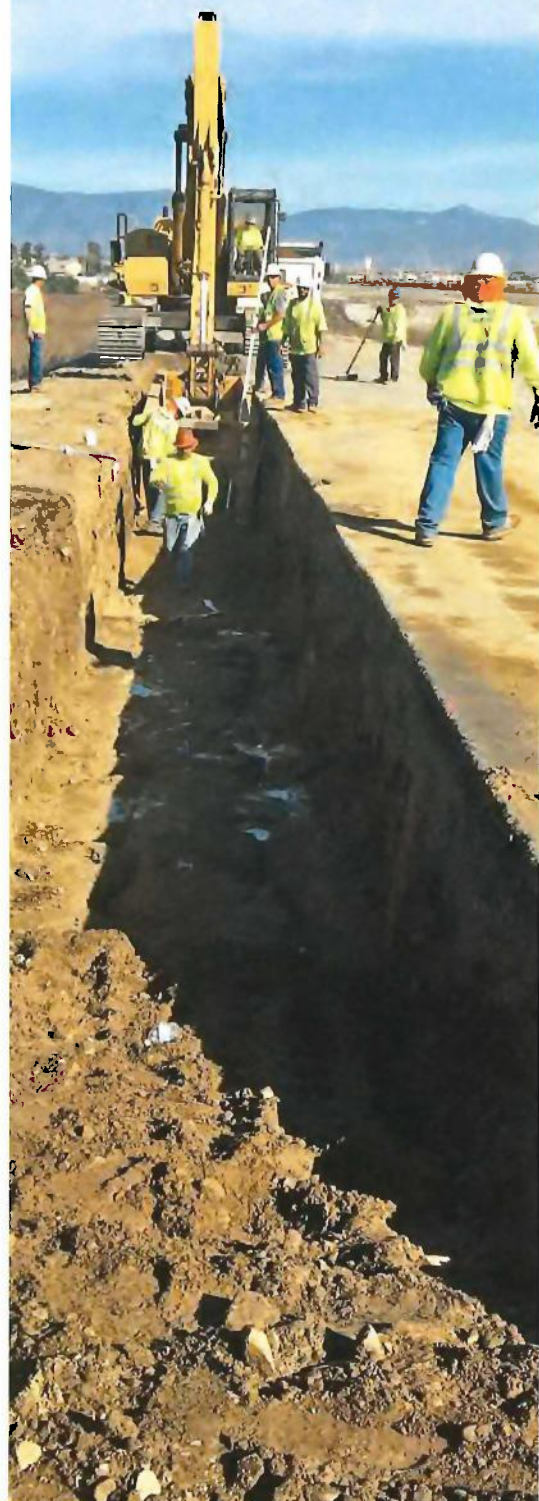
Trenching for pipelines to connect recharge basins.
