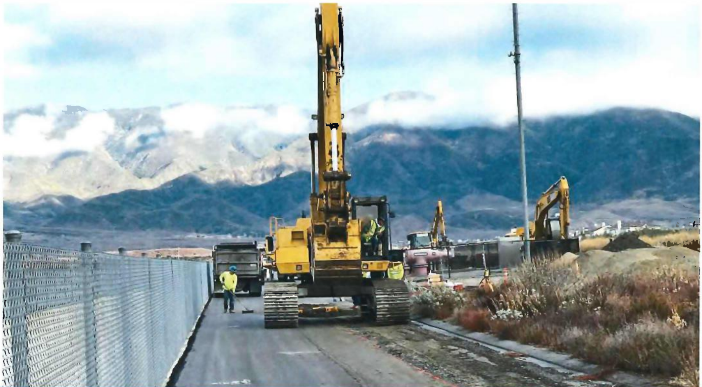
Heavy equipment at work on San Sevaine Basin.
