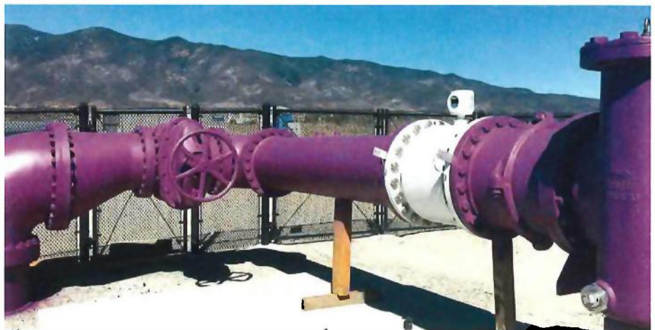
Recycled water pipes and valves being installed to deliver recharge water to San Sevaine Basin.
