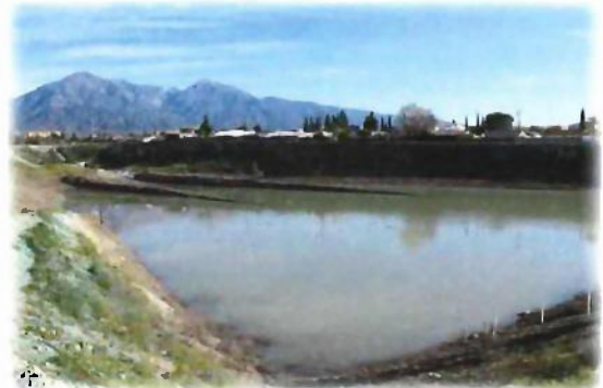
Montclair 1 Basin after a rain storm.
