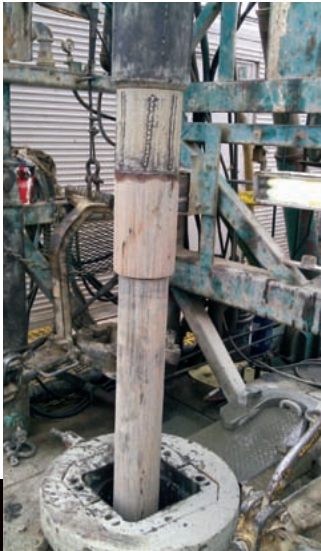
View of a desalter well being drilled.
